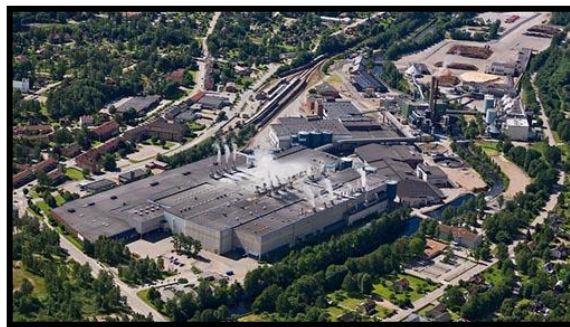
A helicopter view of the plant
